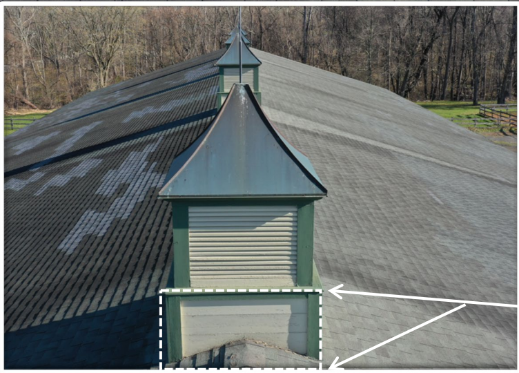
Cover Cupolas below the louver line with Azek board
