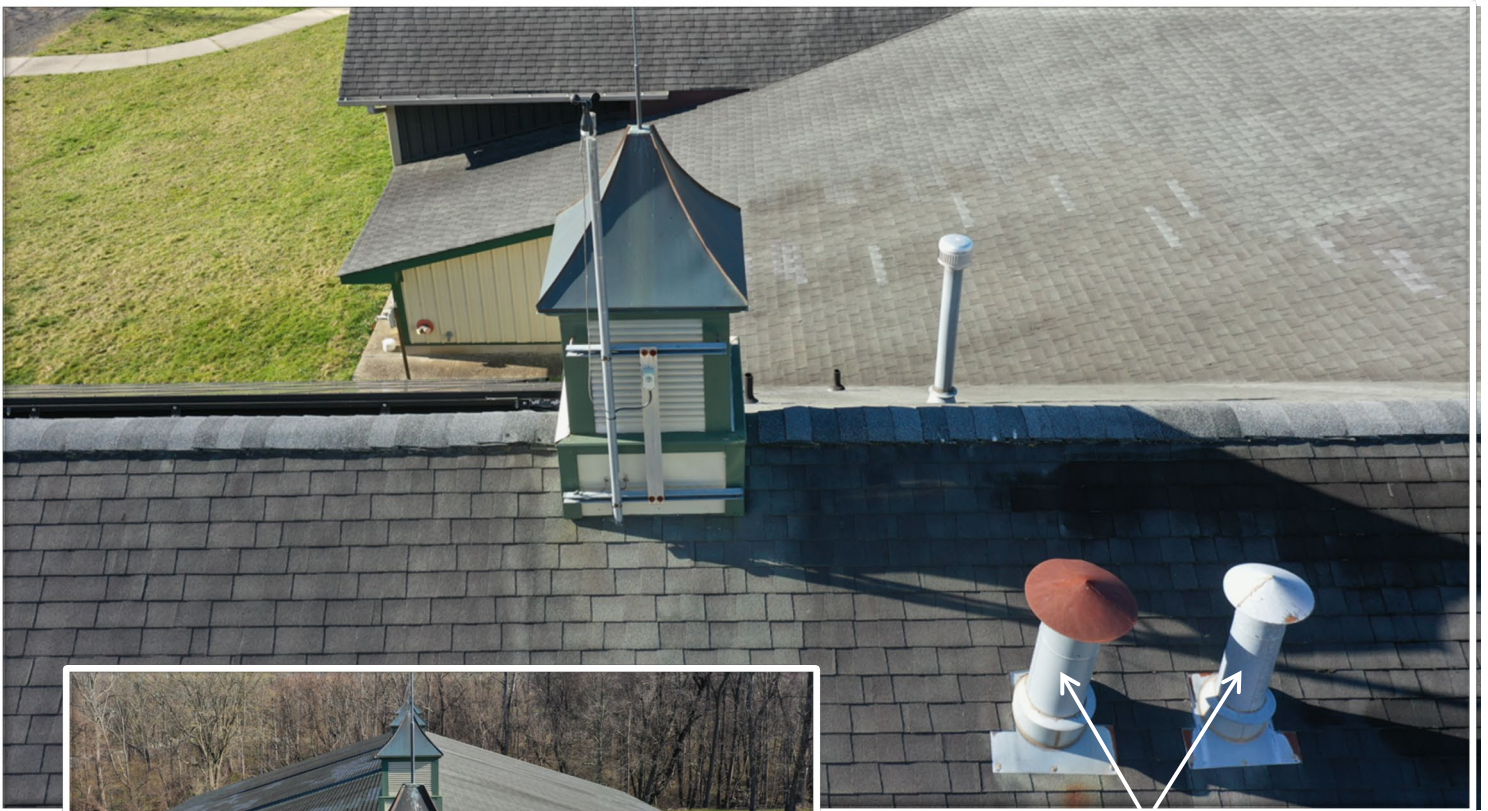
Replace Mechanical pipes below the roof line
