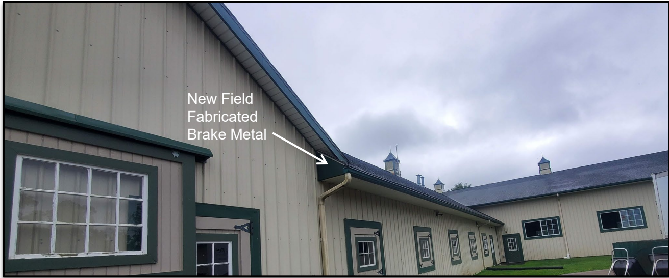
New Field Fabricated Brake Metal
